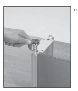
• Finish tightening the lock nut on the gallery post. If there is a glass panel be sure not to over tighten as it will force the bracket down onto the glass causing the corners to crack.
