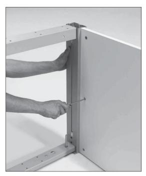
• Turn the mini-fix cam clockwise to tighten modesty panel to the base.
